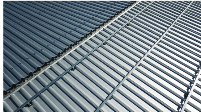
RL LINER DECK DURING INSTALLATION PROCESS
