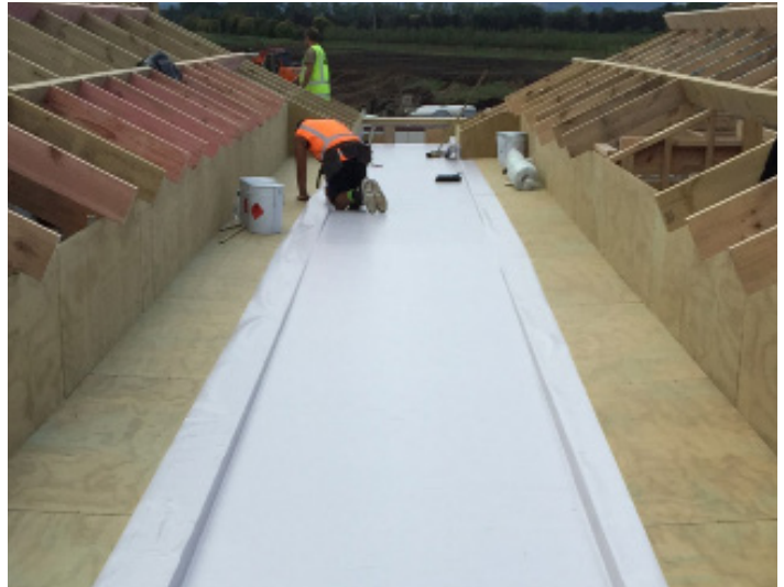
Rooflogic Fibertite SM being adhered to plywood gutters with RL 190EHT.
