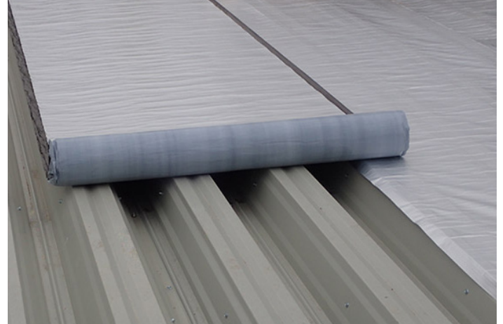
RL Vapour Control Layer being installed over Base Deck
