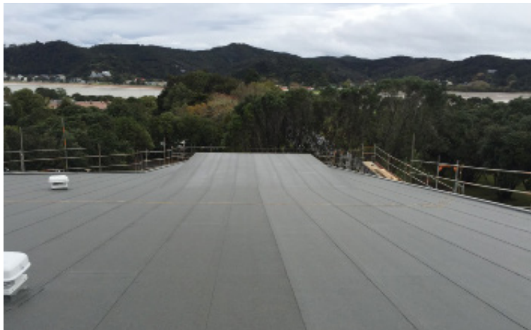
Rooflogic Ultratherm Xtreme with Derbigum System installed to Waitangi Museum, Auckland
