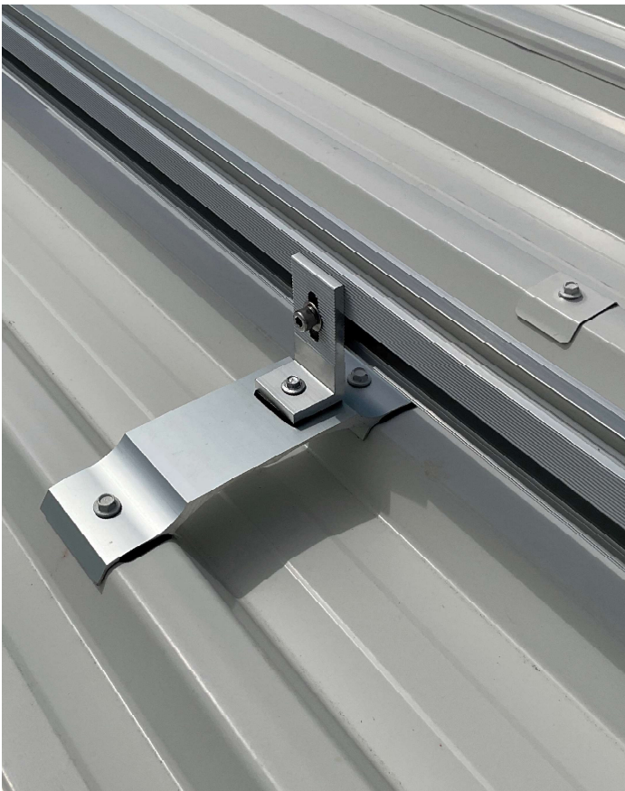
Helios Bracket supporting components for PV array during installation
