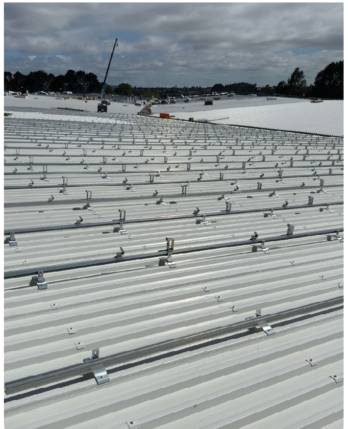
Helios Bracket supporting components for PV array during installation
