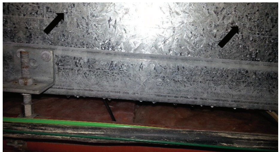
FIGURE 6. Droplet formation on the steel purlin and rust evident on services bolt and nut.
