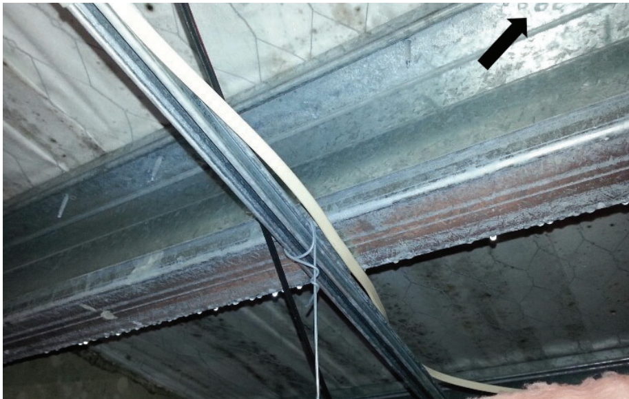
FIGURE 4. Condensate forming on purlins.
