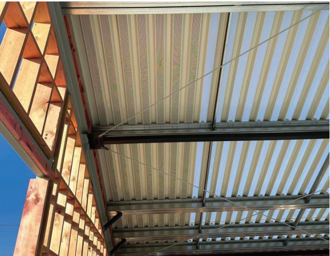
RL Perforated LinerDeck during installation
