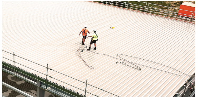
RL LinerDeck during installation
