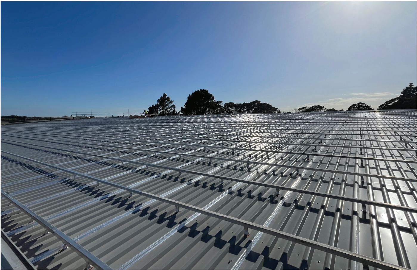
RL LinerDeck with Post & Rails during installation
