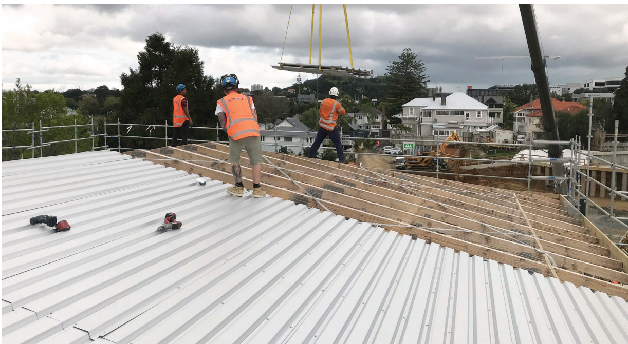
RL BaseDeck exposed with Skylights
