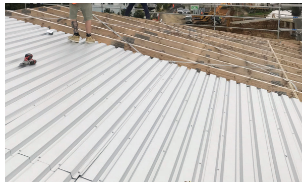
RL BaseDeck running perpendicular to roof fall
