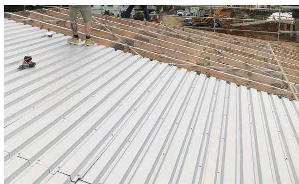
RL BaseDeck running perpendicular to roof fall
