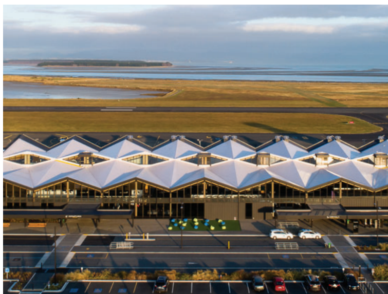
RoofLogic Fleece-Backed Membrane installed over Nelson Airport.
