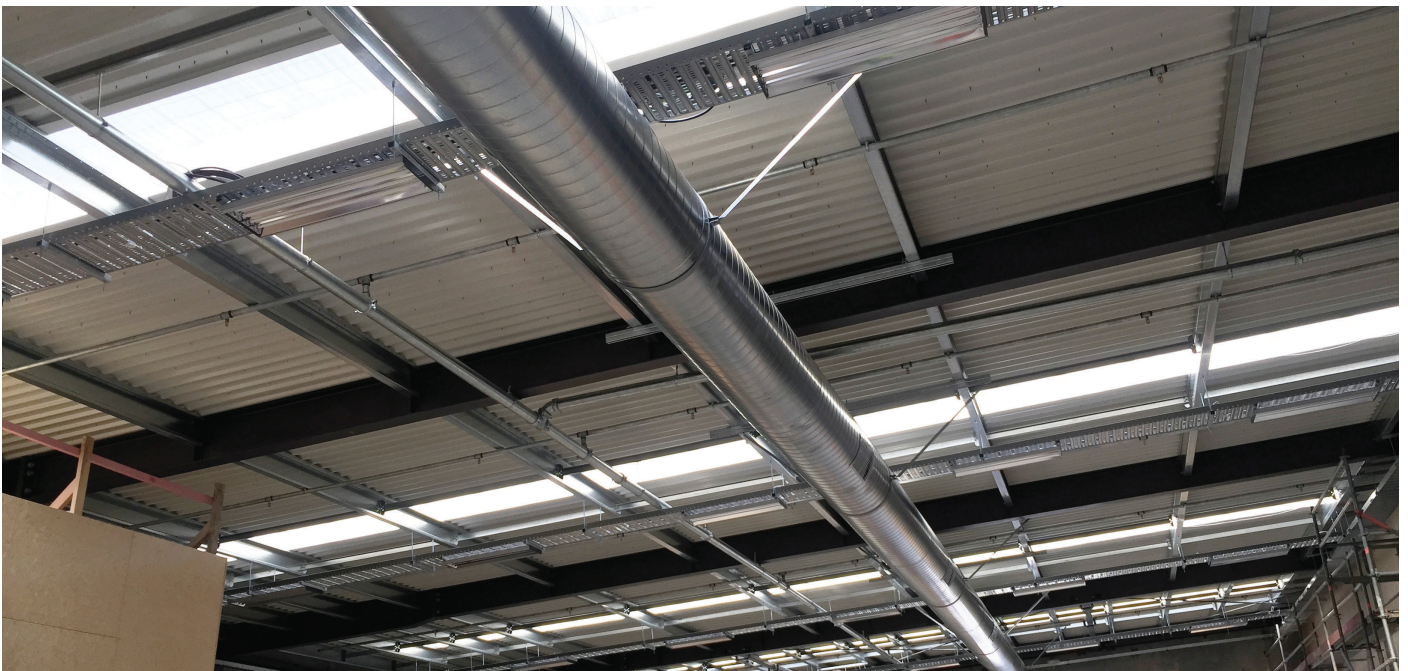
RL BaseDeck exposed with Skylights
