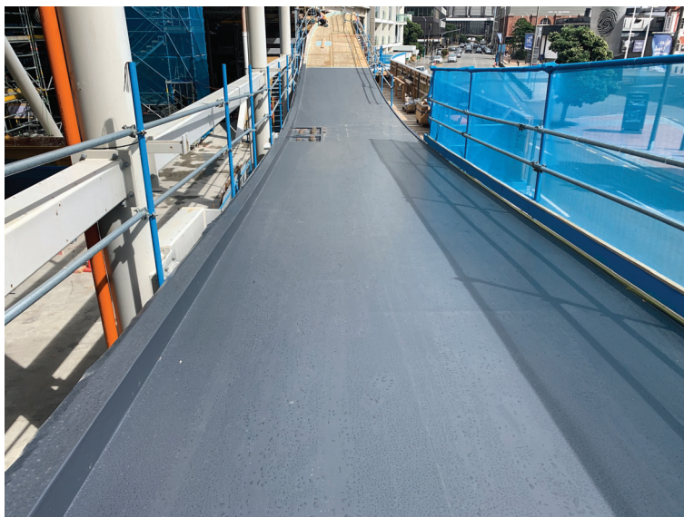
RoofLogic FiberTite SM being adhered to plywood canopy.
