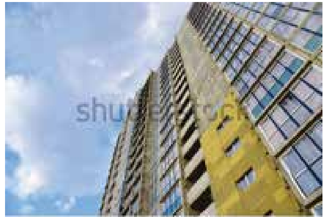
Masonry with rendered insulation
