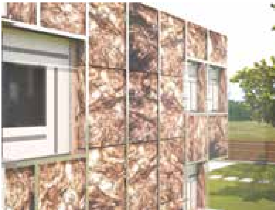
Lightweight structures with glass wool insulation
